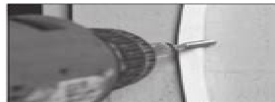
(Fig. 1-4) Connected to temporarily secure door unit.
